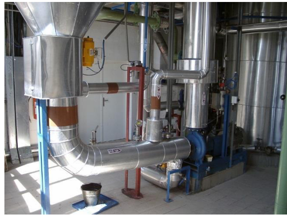
150 t/d loop interesterification plant located in Slovakia
